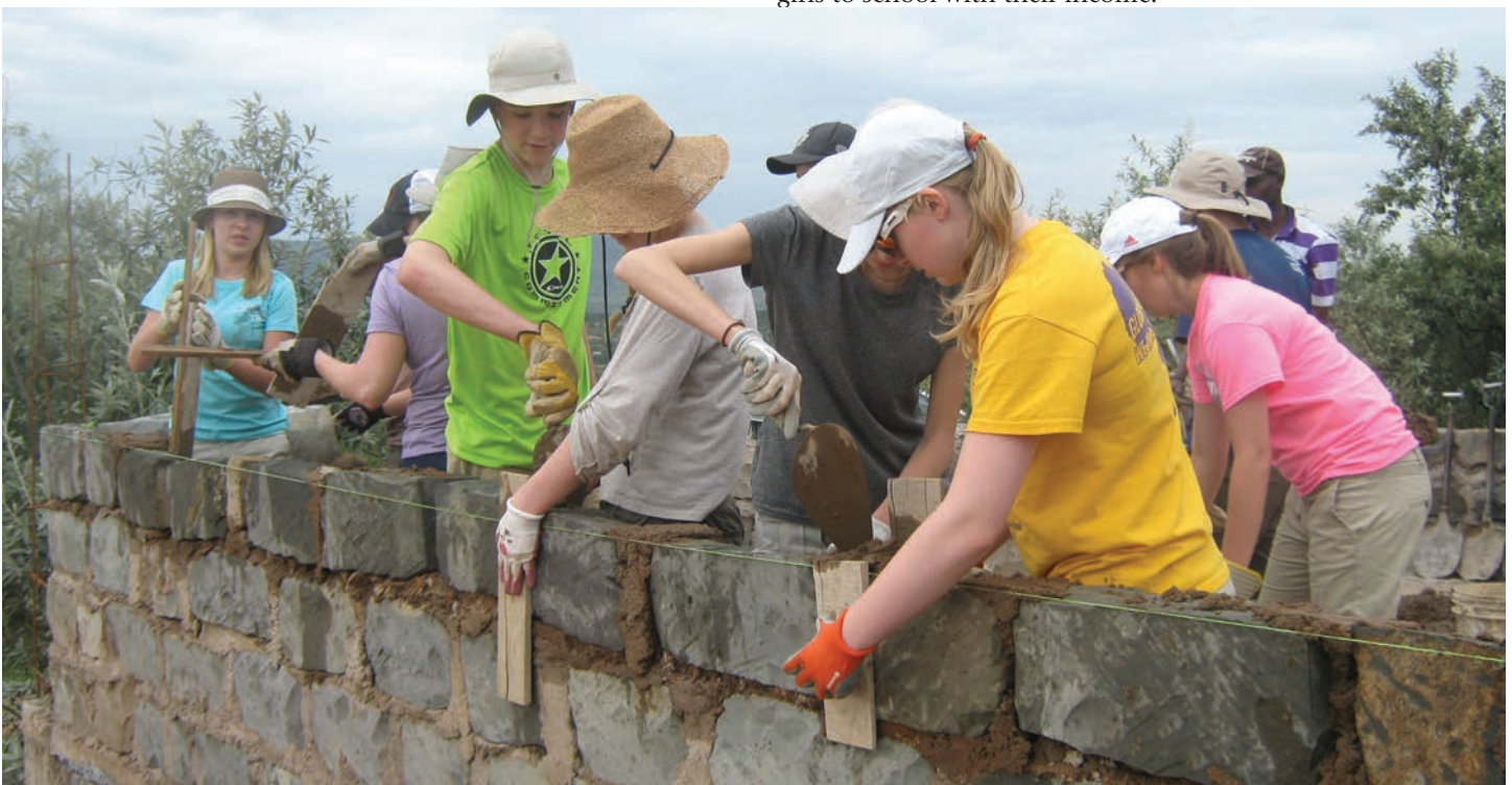
A morning of building the Oleleshwa school in Kenya.
